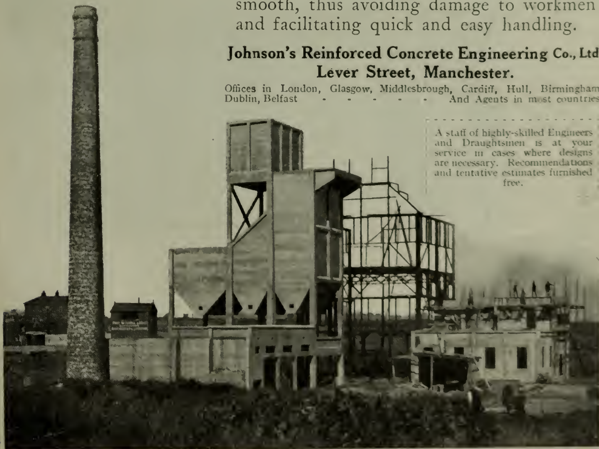
Tank and Coke and Breeze Bunkers erected with Lattice and Keedon Reinforcement for the Gas Department, Scunthorpe Urban District Council. Engineer: S. Moore, Scunthorpe. Contractors: F. Mitchell & Son, Ltd., Manchester.
